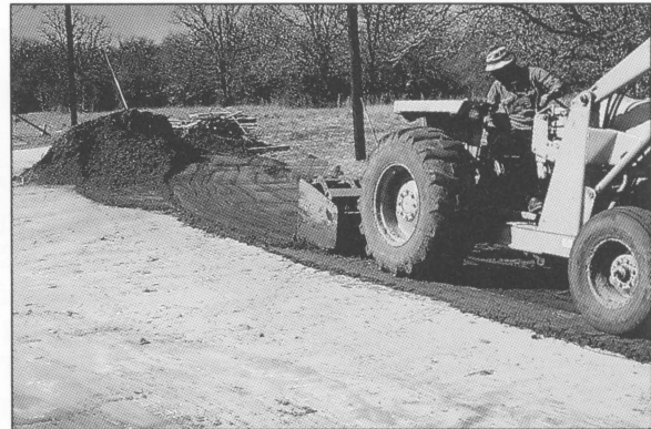
Step 2. Add top soil where needed to fill and provide surface drainage.
