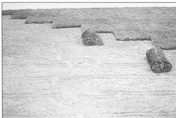
Step 5. Lay sod like bricks on smooth, firm seedbed.
