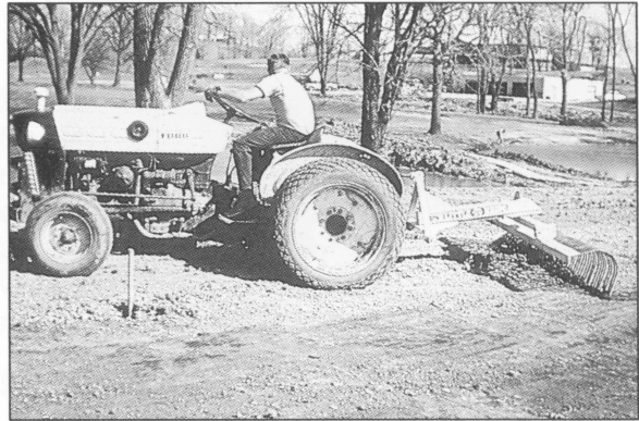
Step 1. Remove rocks and construction debris from the site.
