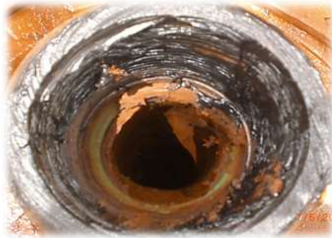
Fig. 1—Deposit and scale in drill pipe (Al-Muhailan et al. 2014).
