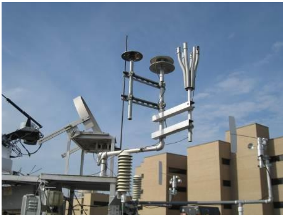
Figure 88. Holding seat structure installed for PSP
