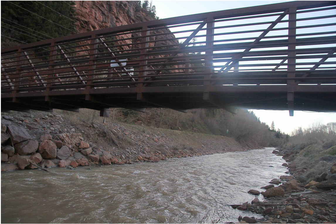
Fig. 36. Looking west at R3 in September 2011.
