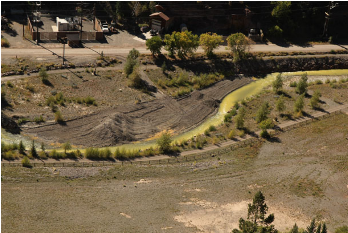
Fig. 39. Oblique aerial image of R2 captured in September 2010 just before artificial bar was removed by the City of Ouray.
