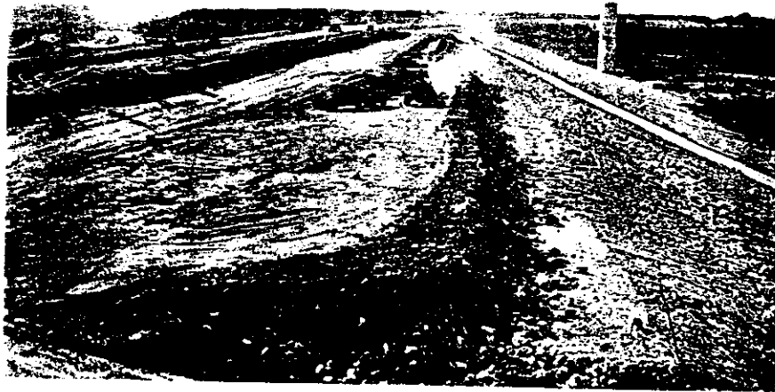
CONSTRUCTION STAGE, EARTHEN DAM, LAKE BELTON, TEXAS, 1953 (Source: Corps of Engineers, U. S. Army, Fort Worth, Texas)
