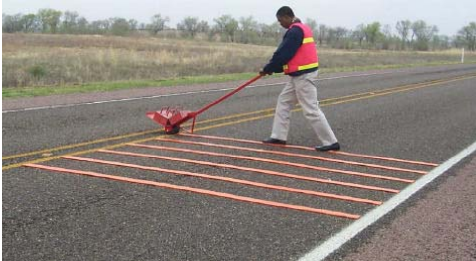
Figure 5 Temporary transverse rumble strips.
