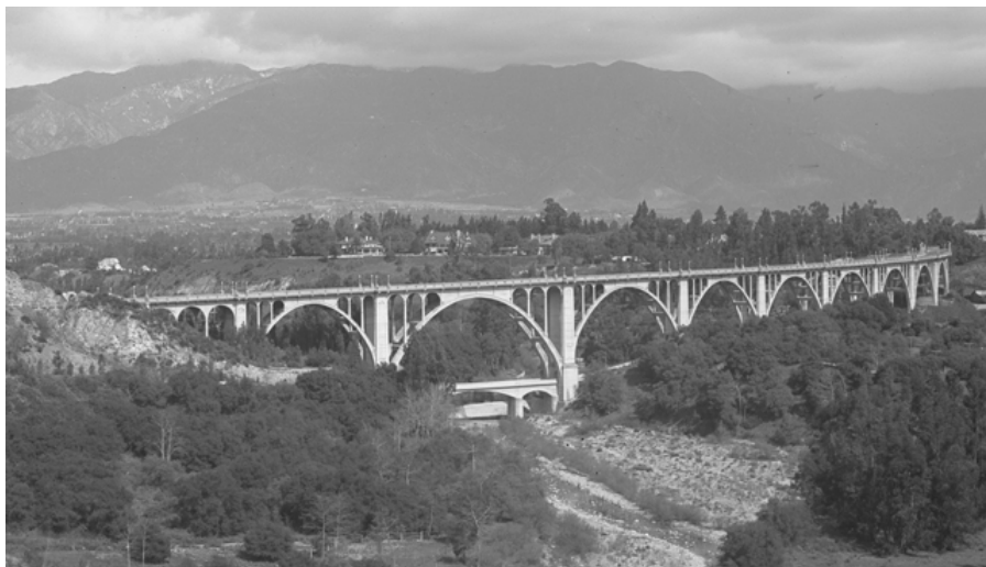
Figure 1.3 Colorado Street Bridge over Arroyo-Seco in Pasadena, California.
