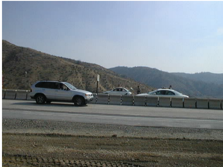
Fig. 14. Movable barrier system separating traffic lanes
