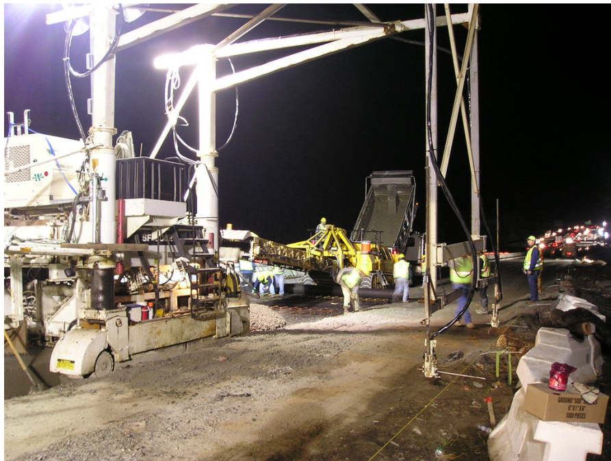
Fig. 19. Paving operations on the I-85 project
