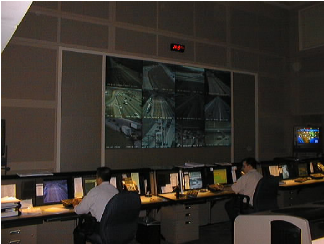
Fig. 23. Traffic management center for the City of Nashville
