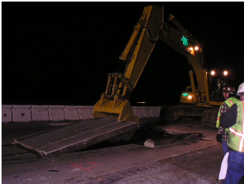
Fig. 18. Removing the pre-sawed slabs with an excavator
