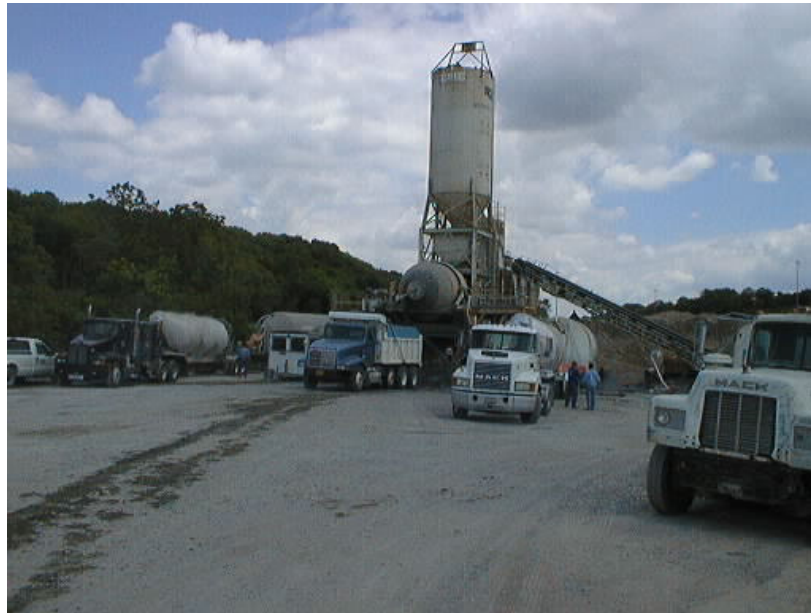
Fig. 22. Exclusive on-site batch plant located near the contractor's office
