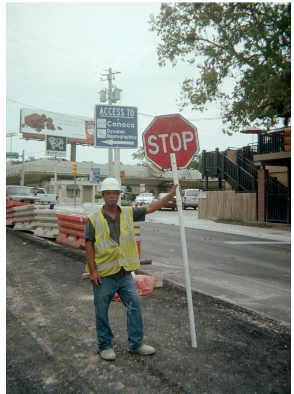
Fig. 8. Access to businesses signing with a flagger to direct traffic
