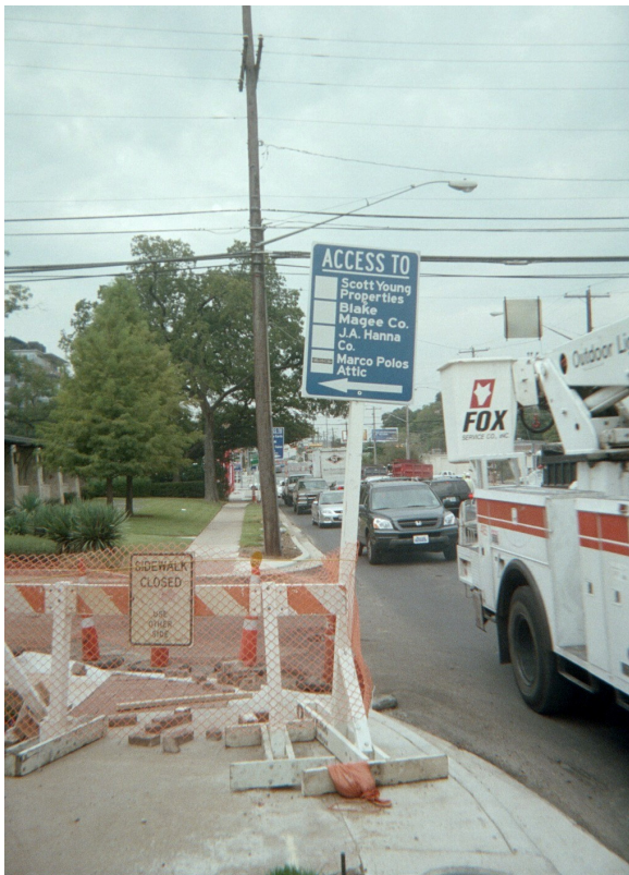
Fig. 7. Business access signs
