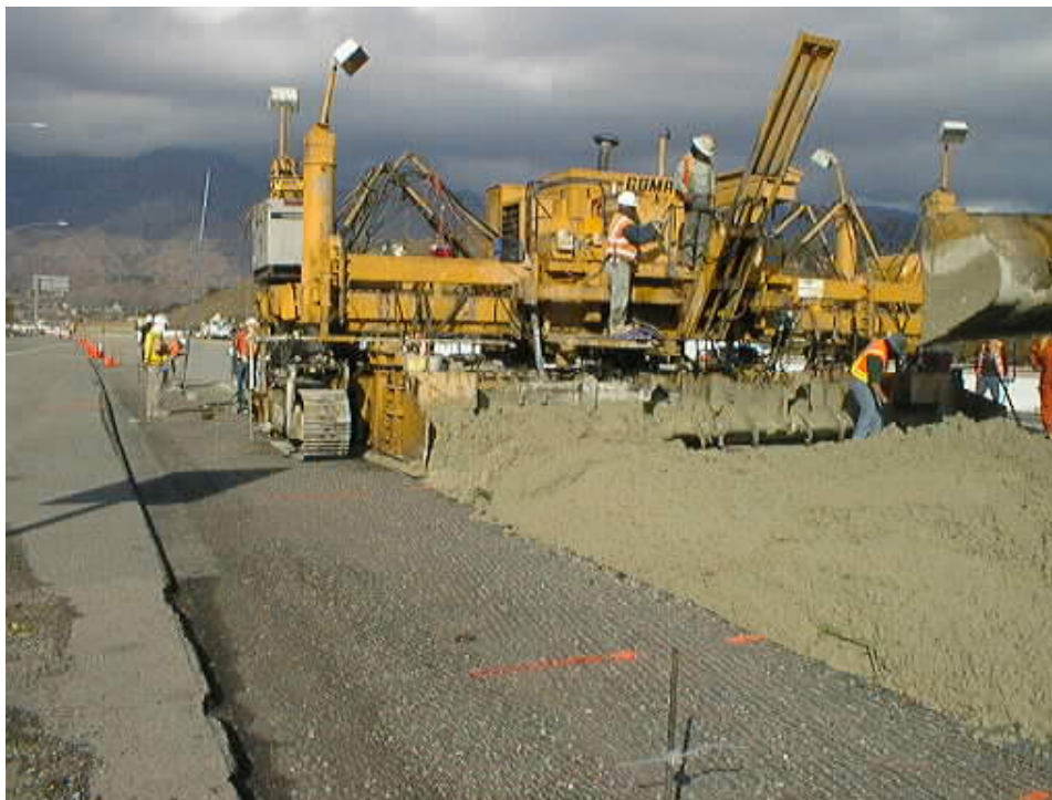
Fig. 13. Paving with a two lane slip-form paver
