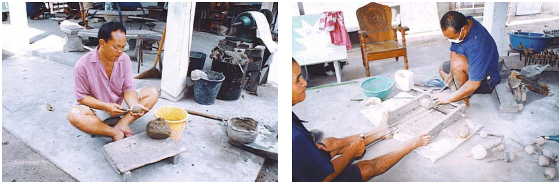
Figure A-8. Constructing the inner mould.
