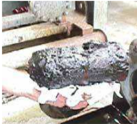
Fig. 2. Deposits removed from a pipeline [2]
