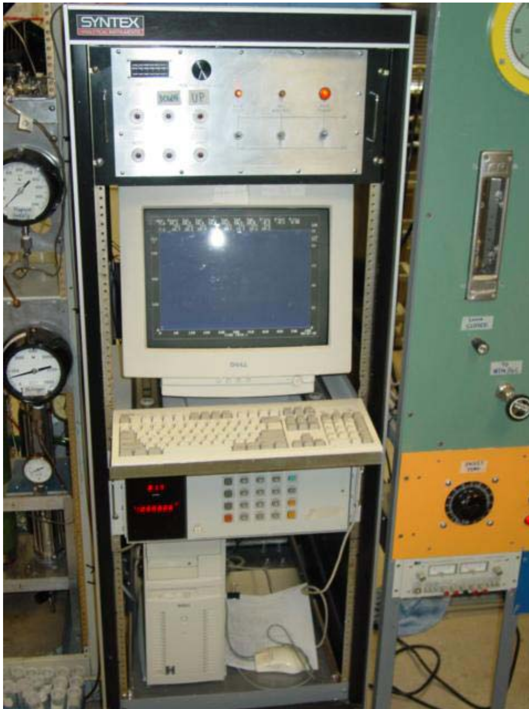
Fig. 3.11—Data logger and PC.
