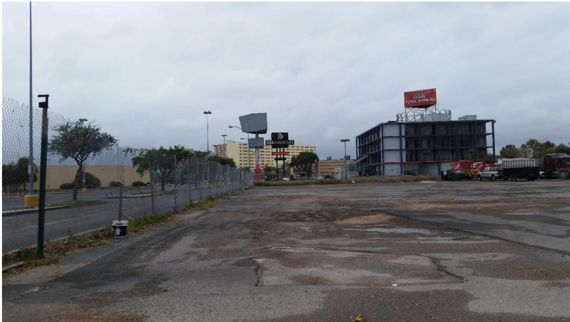
Figure 55: PlazAmericas repurposed and semi-abandoned outlot buildings. SOURCE: G. Marinic
