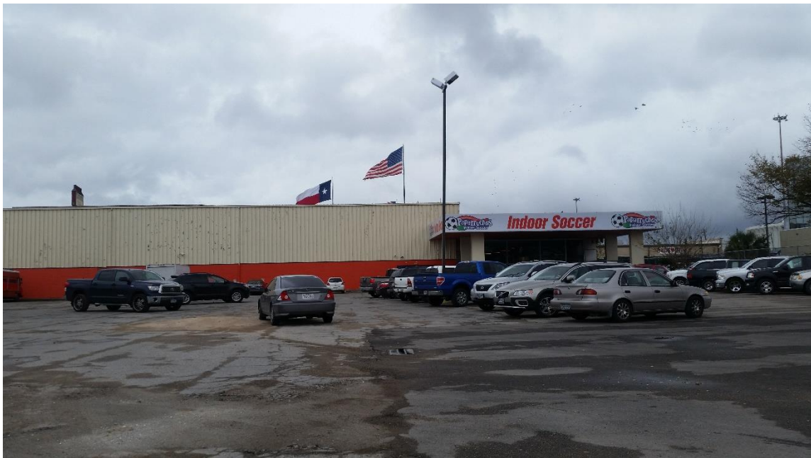
Figure 56: PlazAmericas repurposed and semi-abandoned outlot buildings. SOURCE: G. Marinic
