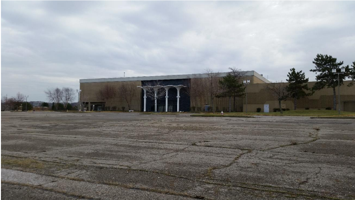
Figure 32: The abandoned Higbee's store at Euclid Square Mall, March 2017. SOURCE: G. Marinic
