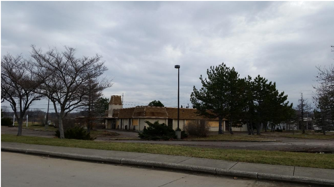
Figure 35: Abandoned outlot building at Euclid Square Mall, former Red Lobster restaurant, March 2017. SOURCE: G. Marinic
