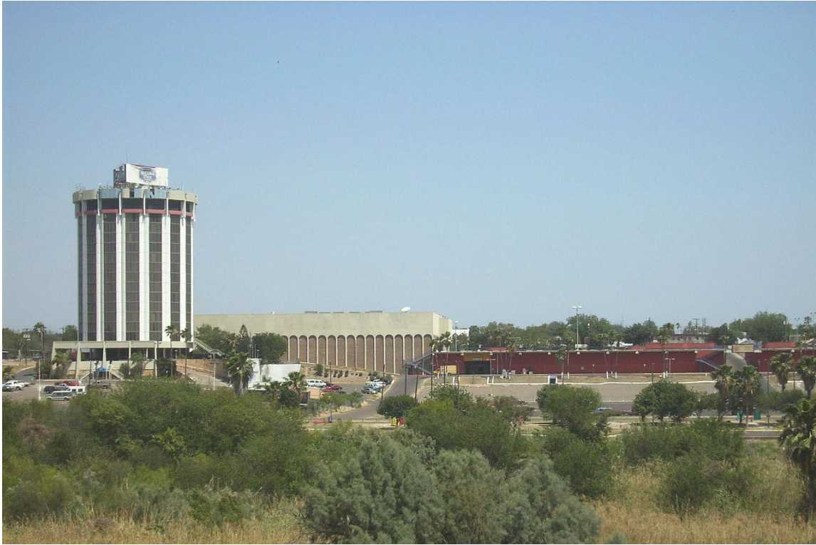
Figure 19: View of River Drive Mall from Nuevo Laredo, Mexico. SOURCE: Wikimedia
