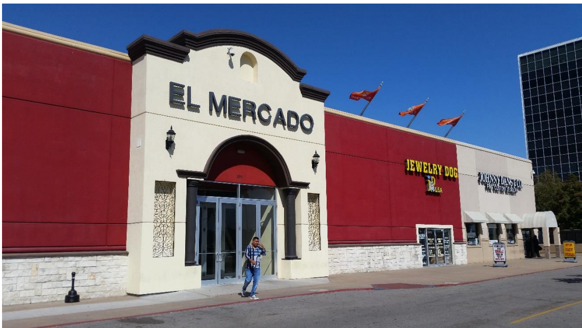
Figure 48: PlazAmericas exterior façades. SOURCE: G. Marinic
