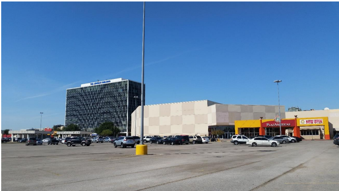
Figure 47: PlazAmericas exterior façades. SOURCE: G. Marinic
