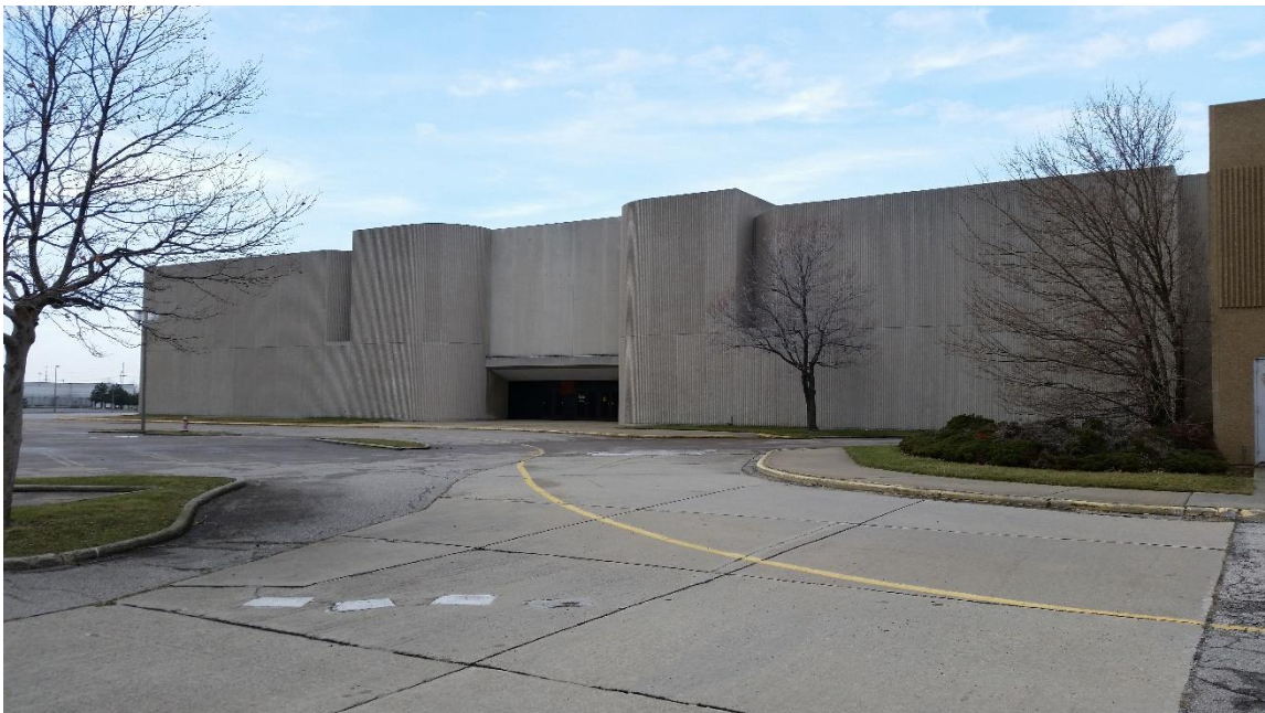
Figure 33: The abandoned May Company store at Euclid Square Mall, March 2017. SOURCE: G. Marinic
