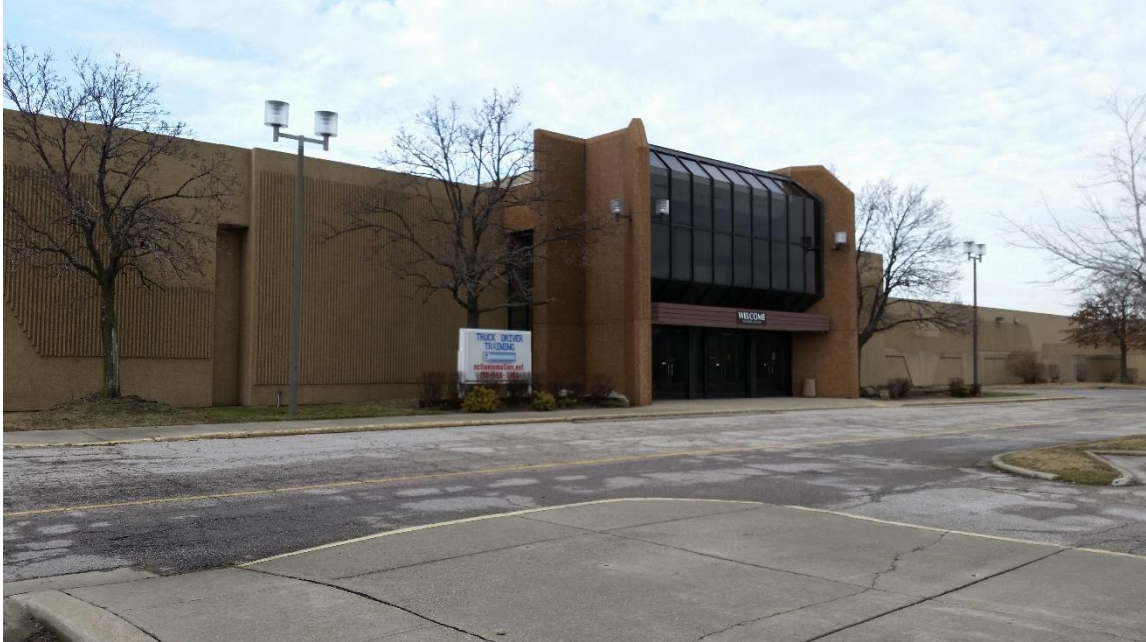
Figure 31: The abandoned Euclid Square Mall, March 2017. SOURCE: G. Marinic
