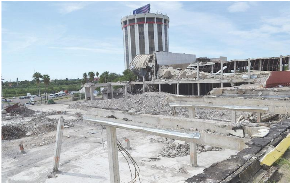
Figure 21: Demolition of River Drive Mall in mid-2015. SOURCE: Alberto Carrasco
