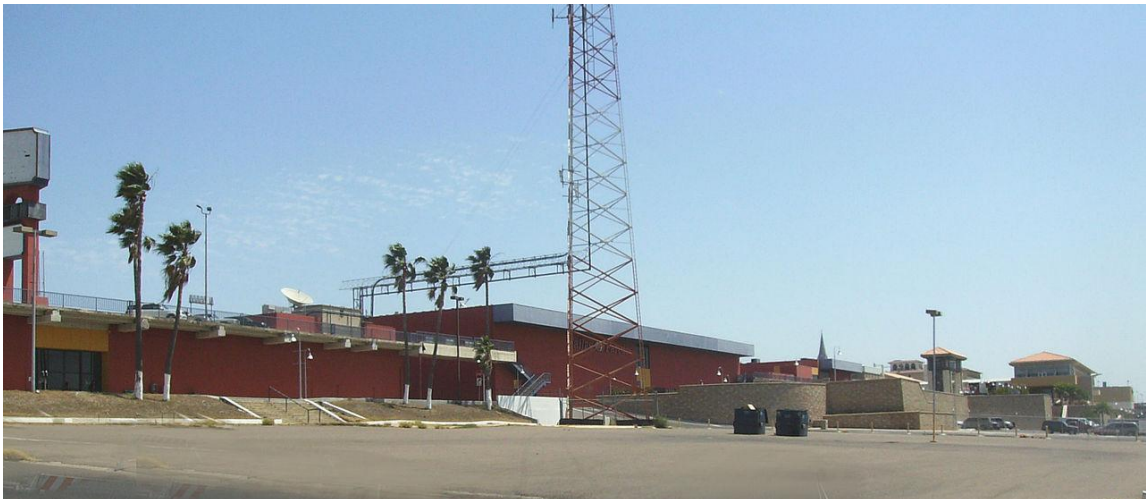
Figure 20: View of River Drive Mall. SOURCE: Wikimedia
