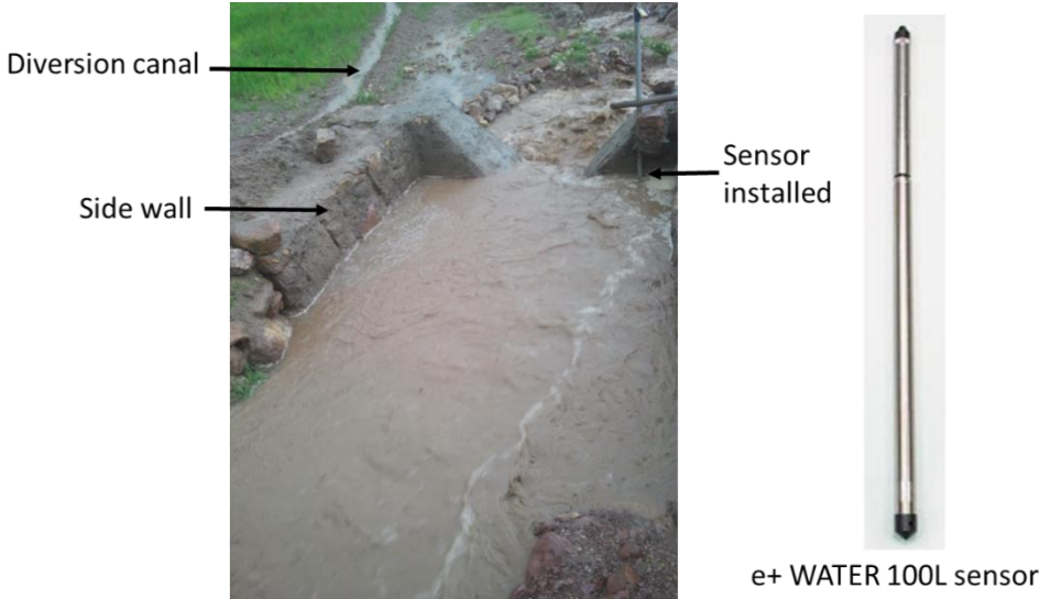
Figure 4.4 V-notch, diversion canal, side wall, sensor and runoff in gully reach in sands stone (S).
