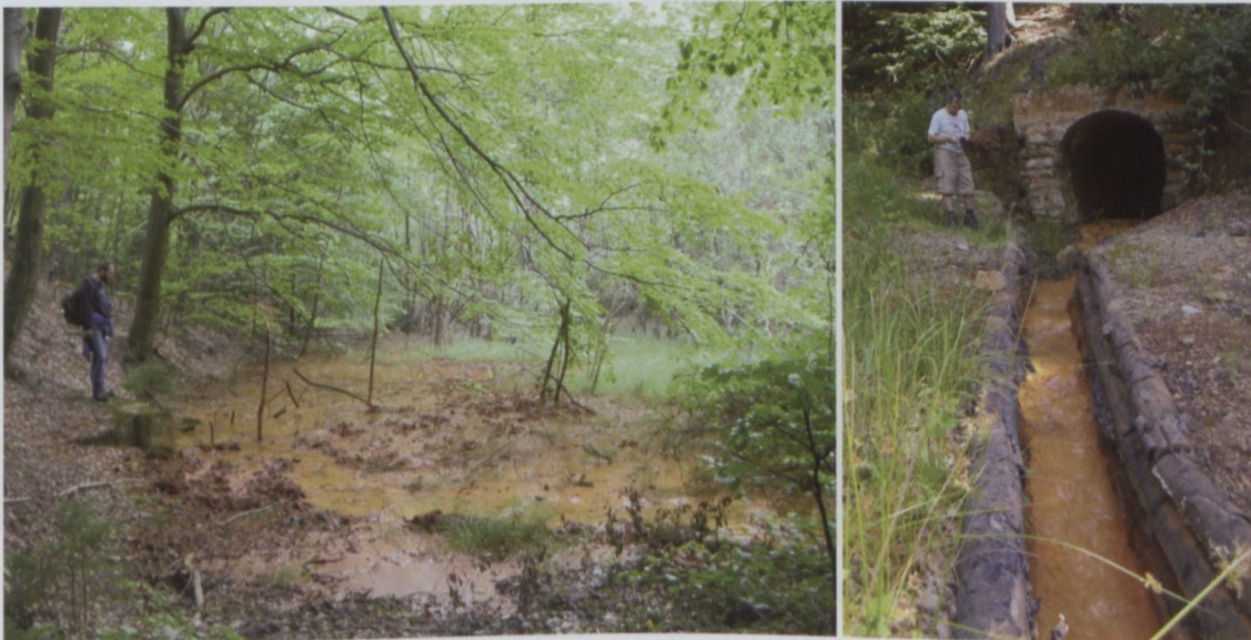
Fig. 25. Collar of Anna-Agnes adit at Poproč prior to and after remediation.
