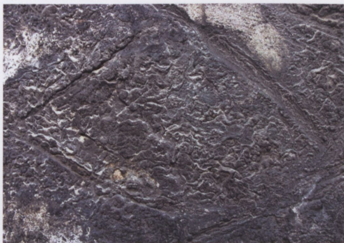
Fig. B4. Folded surface of black gypsum crust on the Upper Jurassic limestone; Kraków, City Walls.
