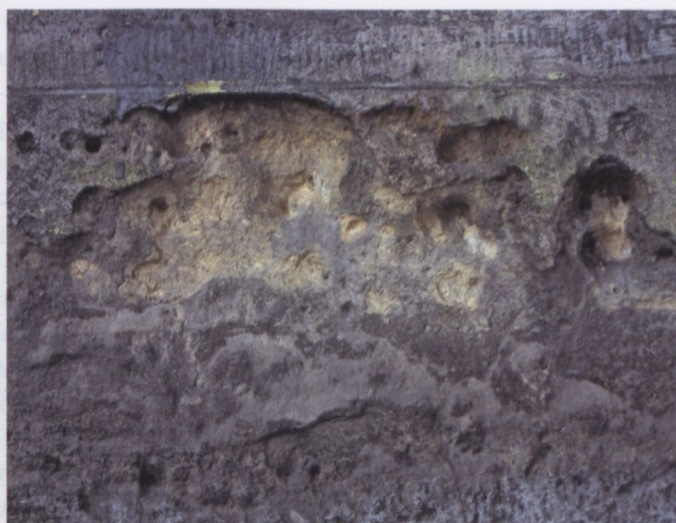
Fig. B12. Alveolae formed during weathering of the Libiąż dolomite. The surface of the rock is partly covered by black gypsum crust.
