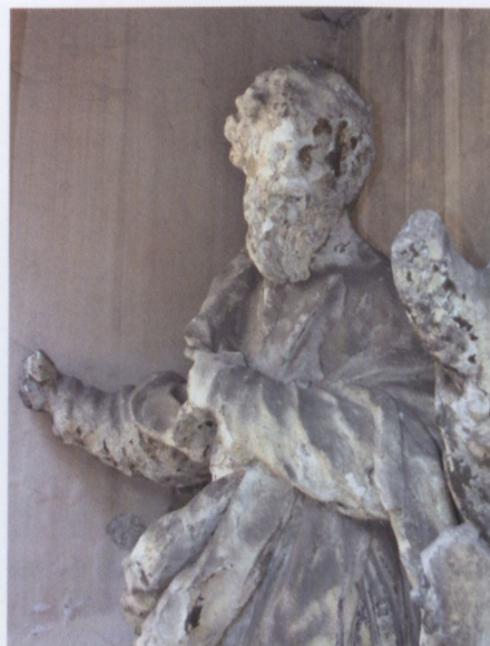
Fig. B7. Deep disintegration of the Pińczów limestone; an Apostel statue from the St. Peter and Paul Church, Kraków. The statue is now sheltered under a roof, which results in deposition of grey dust on the rock surface.
