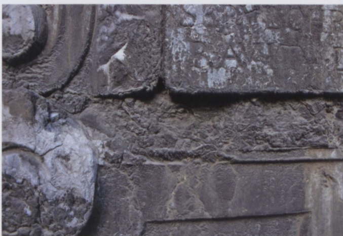
Fig. B11. Black gypsum crust on the Dębnik limestone (folded surface of the gypsum crust); Carmelitan church, Kraków.
