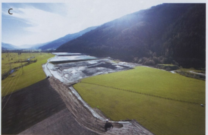
Fig. 19. a) Beneficiation plant 3 km north of the mine, directly at the Felbertauern highway. b) Overview of milling and flotation circuit. c) Tailings management facilities in the Pinzgau valley near Stuhlfelden showing the extent of the re-cultivation measures that occur concurrently with the operation.
