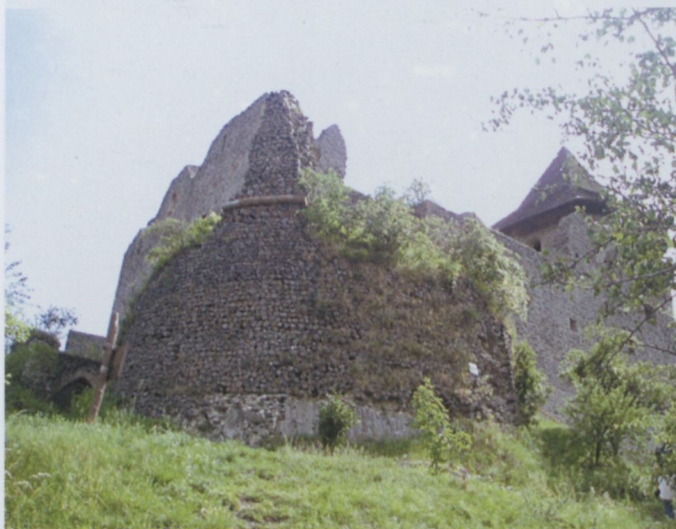
Fig. 17.1. Ruins of medieval Šomoška/Somoskő castle; the walls were built from basalt columns. Photo: P. Uher.
