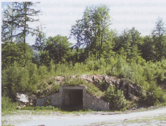
Fig. 14.1. Entrance of the exploration adit in Dlhá dolina valley near Gemerská Poloma. Photo: P. Uher.
