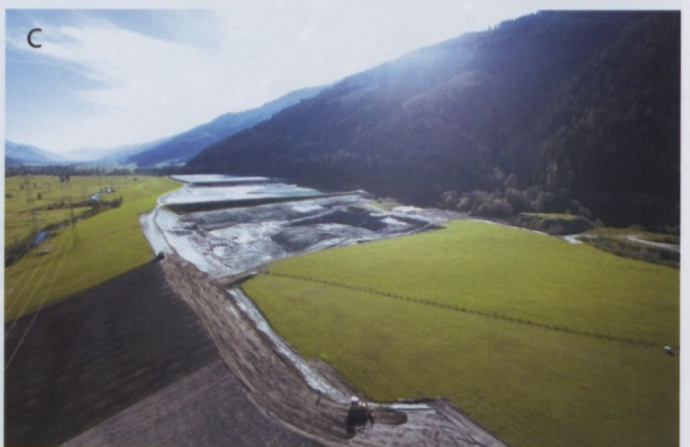
Fig. 19. a) Beneficiation plant 3 km north of the mine, directly at the Felbertauern highway. b) Overview of milling and flotation circuit. c) Tailings management facilities in the Pinzgau valley near Stuhlfelden showing the extent of the re-cultivation measures that occur concurrently with the operation.
