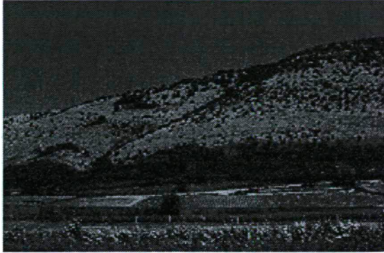
Photo 2 Erosion slope in the Villányi Mountains
