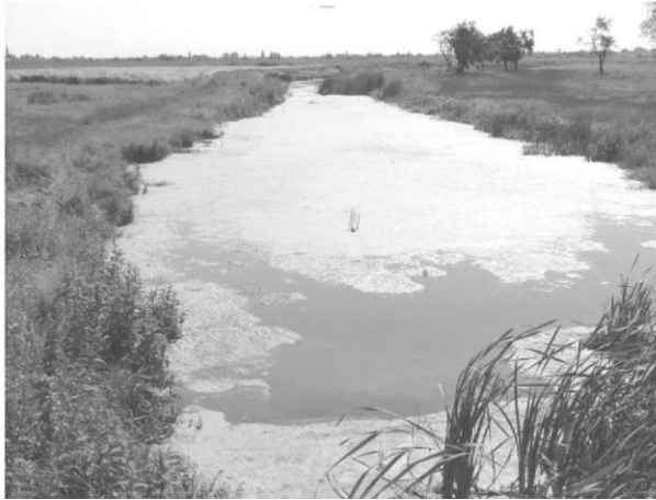
Clogged canal in Bezdin area
