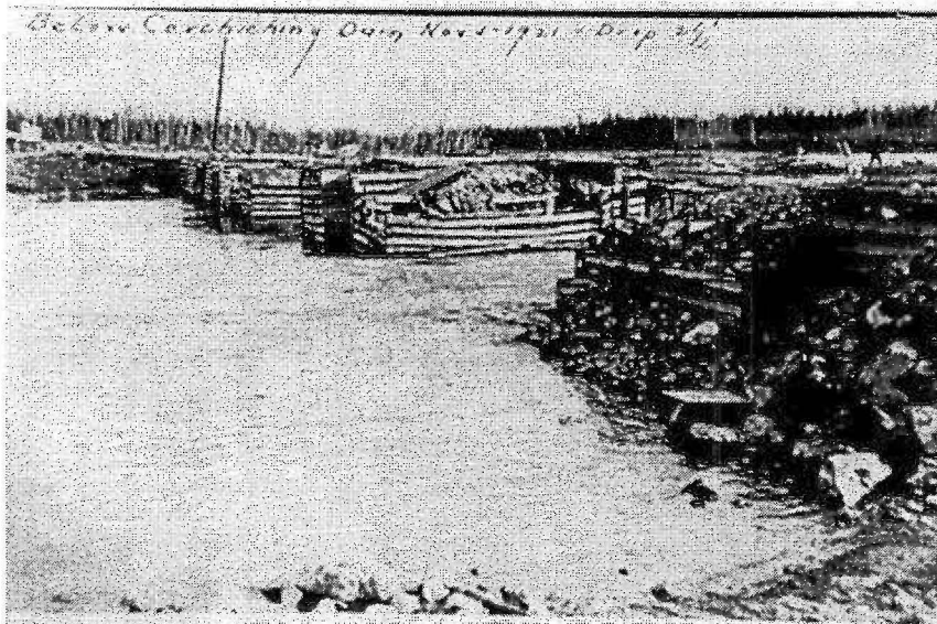
Plate 3.2: The Couch Falls dam on Abitibi River on November 5, 1921. The waters banked-up by the Twin Falls dam have reached but not yet flooded the Couch Falls dam, which is in fairly bad shape just before being submersed. The hand-written note on the upper part indicates that the water dropped about 75 cm (2.5 feet) at this time of the year. (Photographer: H. L. Sanborn)
