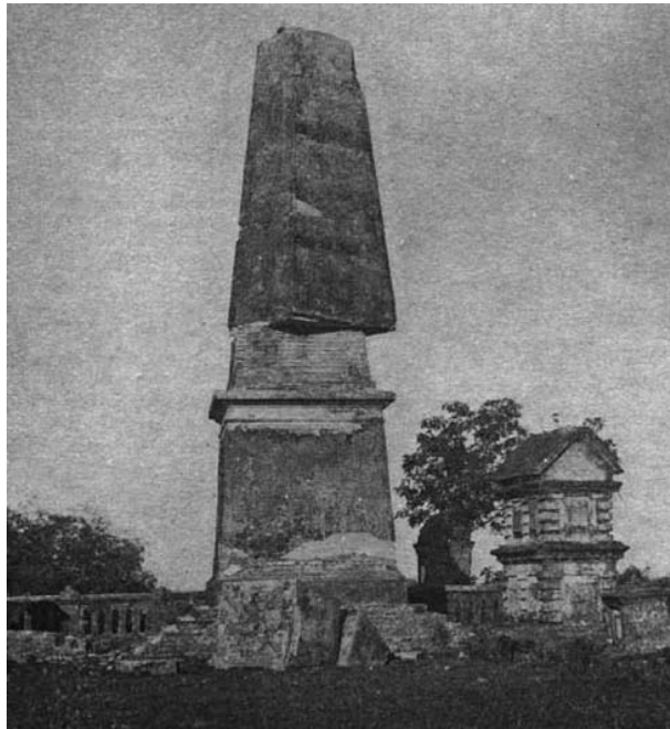
Figure 2.3: Rotation of obelisk segments from the 1897 Assam earthquake (Oldham, 1899).
