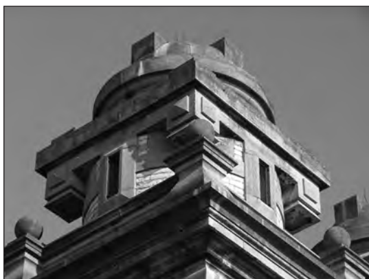
Figure 2 Top of the vertical part with the dome
