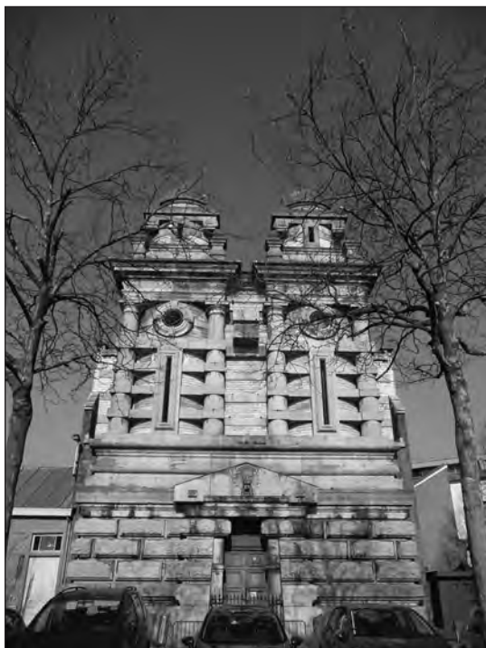
Figure 1 Southern Pressure House: front view
