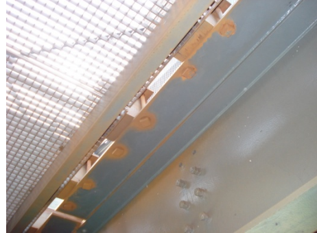
Figure 10: Sleepers-longitudinal girder connection by catch bolts
