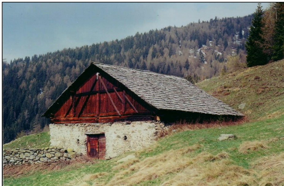
Fig. 3-8 “Maso Cavè”, one of the sampled rural buildings.
