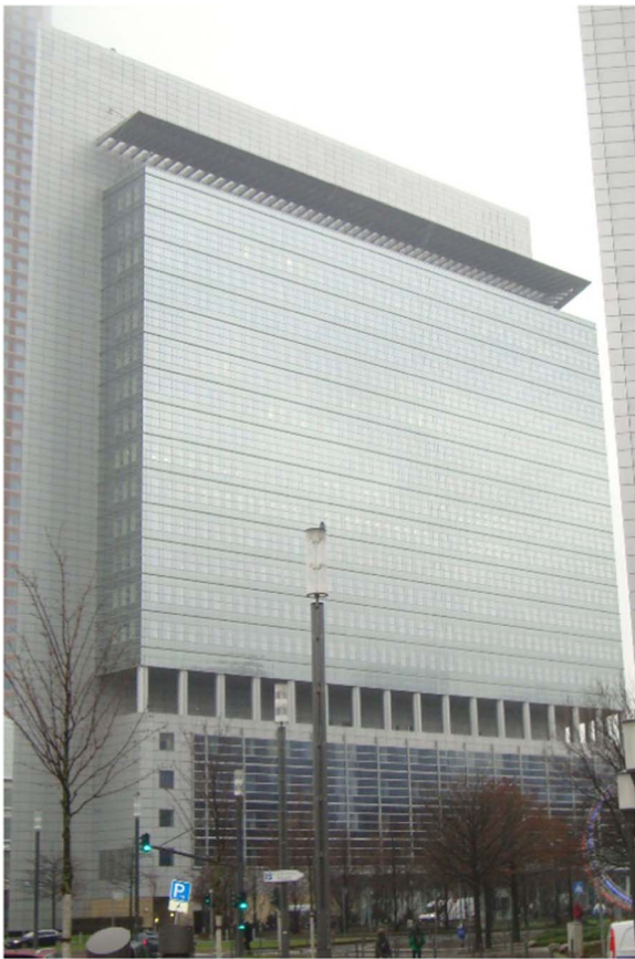
Fig. 1. Example of a two-side supported structural glazing system: Kastor tower in Frankfurt/Main (Germany) [8].
