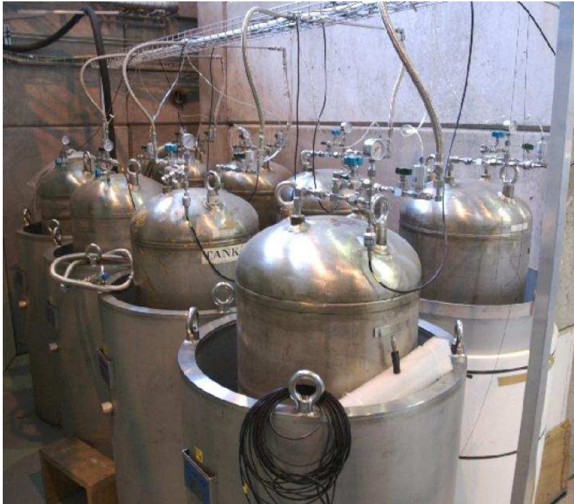
Figure 3.5: Gas xenon storage tanks in the experimental area.
