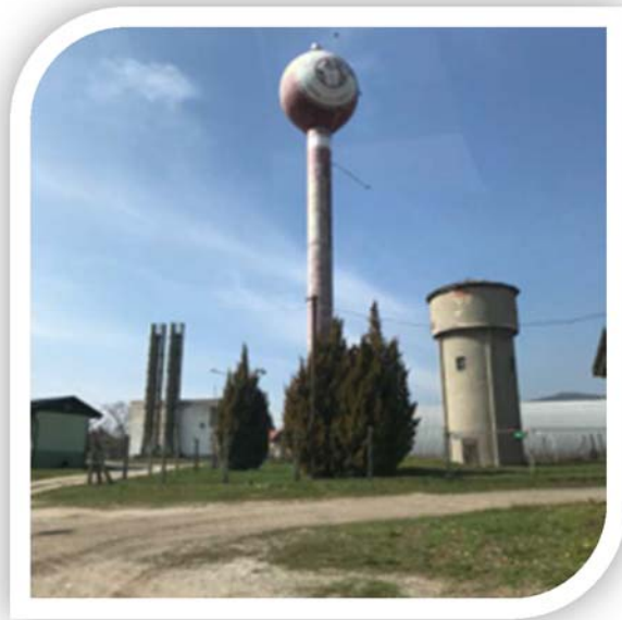
Figure 7 – Water storage tower at the site
