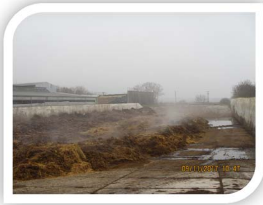
Figure 16 – Manure deposit at the Oponice Plant
