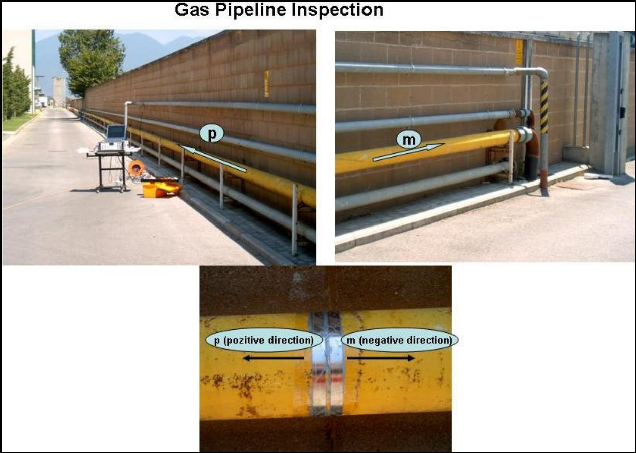
Figure 5-6 Experimental setup for the 6” gas pipeline
