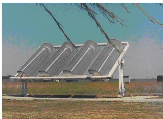
Figura 6 sistema line focus, installati in California( www.entechsolar.com )
