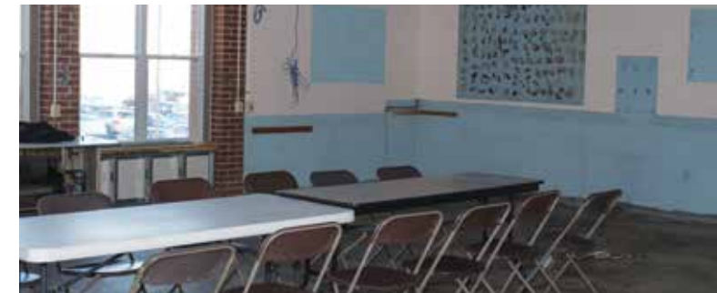
Blewett 108 prior to renovation
