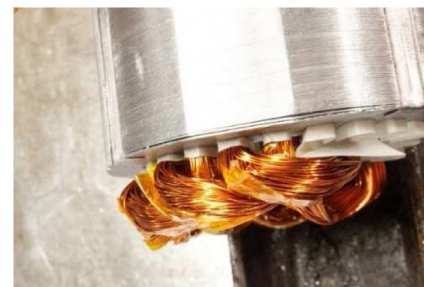
Figure 13. Details of phase to phase insulation during coil insertion
