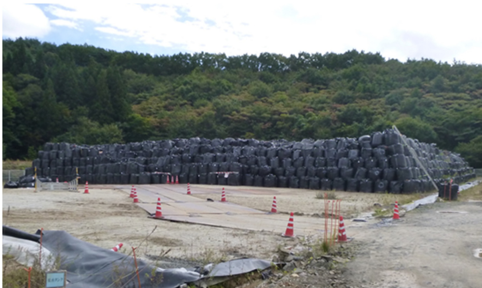
Fig. 1. Photograph of a typical waste storage study site within Kawamata (Date District), Fukushima Prefecture, prior to final waterproofing of the structure.
