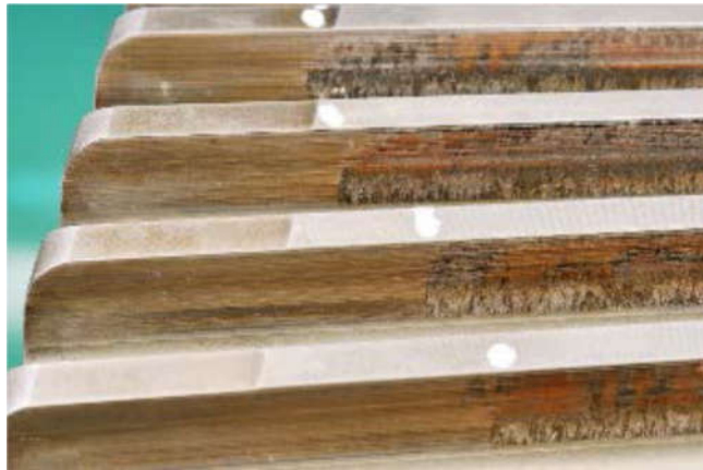
Figure 2.32– scuffing on the high speed stage of wind turbine [107]
