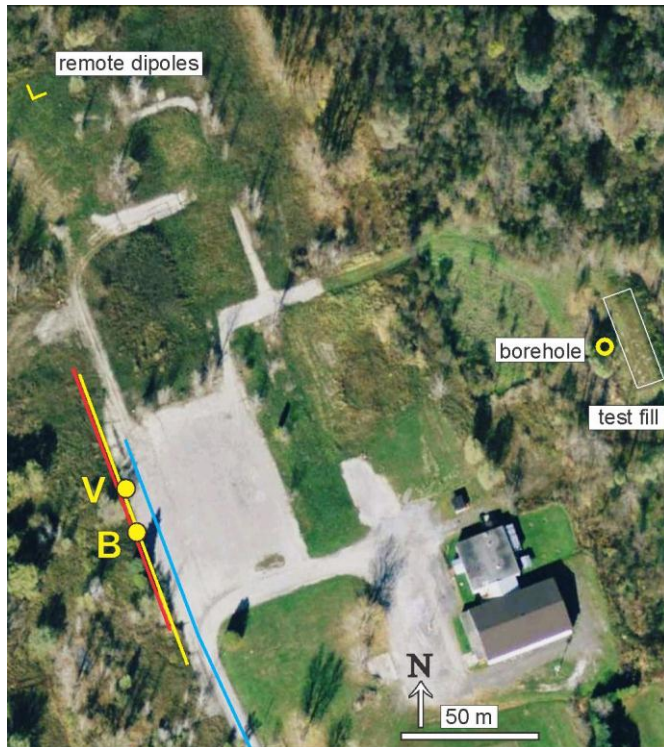
Figure 1. Aerial photo of the study site near Ottawa, showing positions of the seismoelectric recording array (yellow line), the ERT section (red line), the microvibe seismic section (blue line extending 140 m off the map), the remote dipoles, and borehole BH-NRC-MO at the NRC Geotechnical Test Site. Points B and V are the midpoints of supergatherers acquired using buffalo gun and vibroseis sources respectively.
