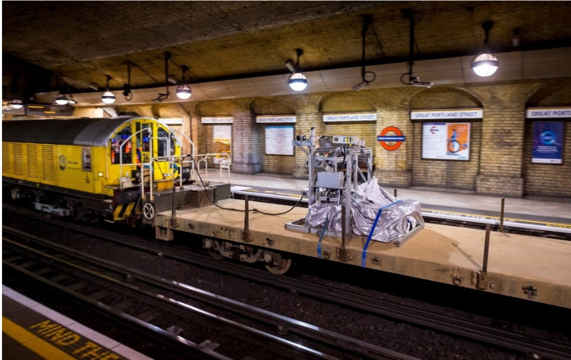
Figure 4. Laser train in use
