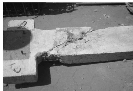
Figure 5 Failure of Specimen C1
