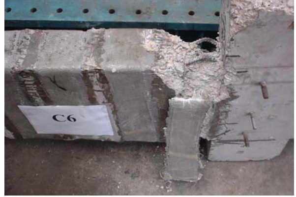
Figure 8 Failure of column C6
