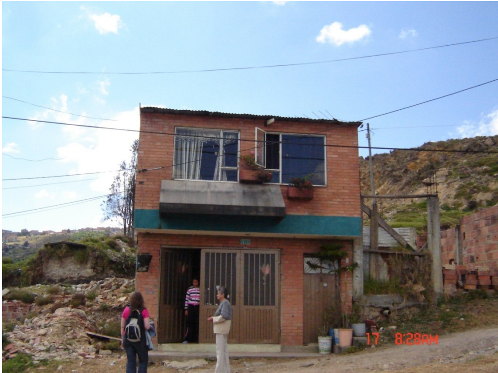
Figure 8: Home owner's house in the San Rafael barrio, Altos de Estancia
