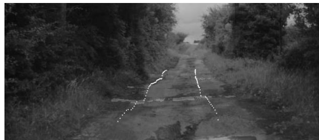
Figure 8.19. Example image from Constructors Road data set.
