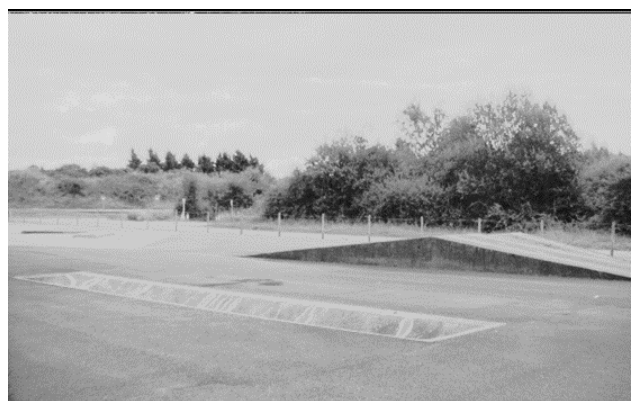
Figure 7.18. Concrete ditch used in experiments
