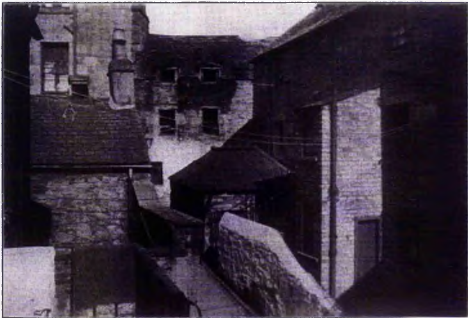
Plate 21: Photographs of slum housing - 'Todburn Lane, East End' and 'Paradise Lane, North East Corner'.
