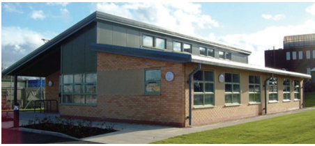
FIGURE 7: Picture of the case building.
