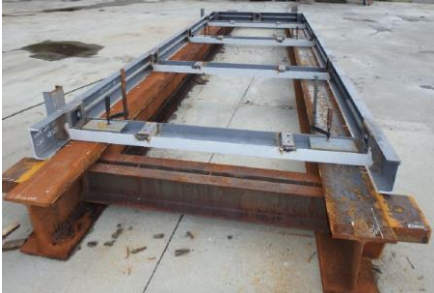
(b) Steel frame (top part)
