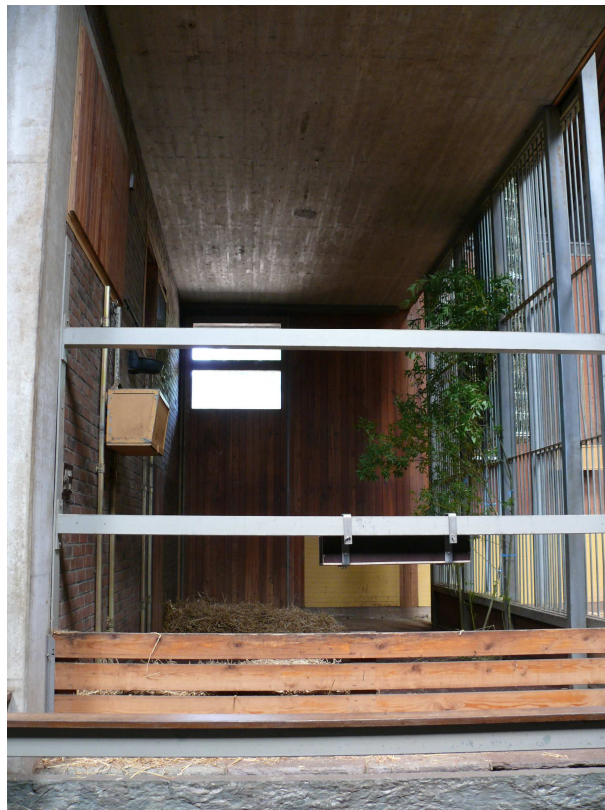
Abb. 3.11: Blick in Box 3 des Kölner Giraffenstalls.
