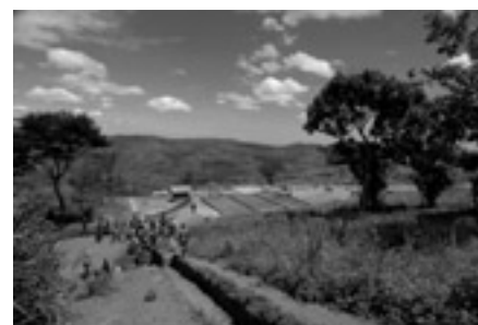
Construction of the GRACE Center Photo: PASA/DFGFI/Disney/MGVP
