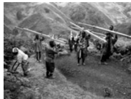
Young people carry material for the construction of the patrol post – 5 hours walking distance!
