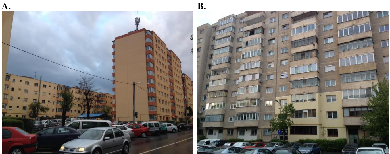
Figure 1: Typical rented social housing in Romania: A. refurbished; B. not refurbished
