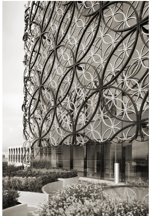
Fig. 12 the facade of the Library of Birmingham designed by Mecanoo, Birmingham, United Kingdom. 2013. Photo: Christian Richters
