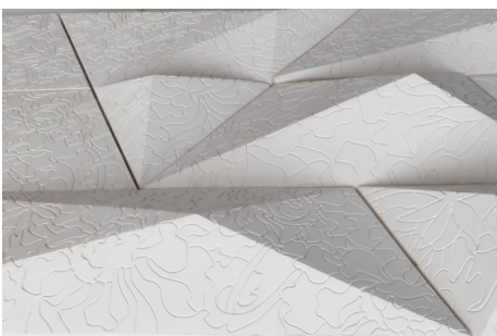
Fig. 38 the ceramic panels on the concert hall in Fuzhou Strait Culture and Art Center. PES-Architects.
