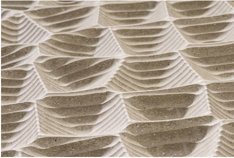
Fig. 34 high-density gypsum fibreboard panels, Elbphilharmonie Hamburg, Herzog & de Meuron.
