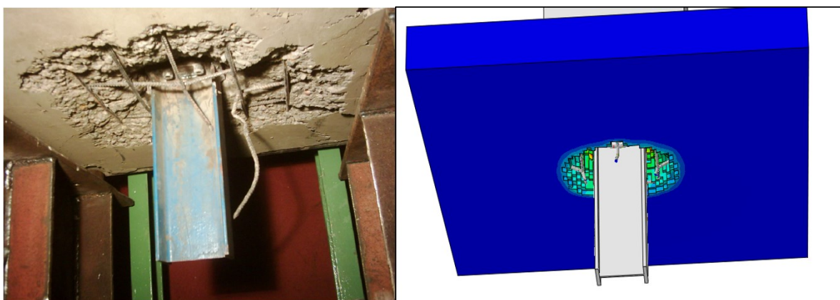
Figure 43 Perforation of I-section into the concrete slab from the experiment and the analysis.
