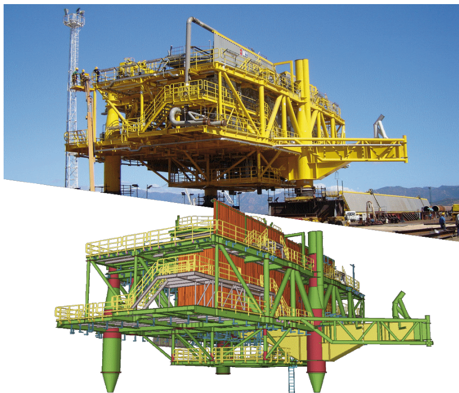
Figure 1: The Halfdan offshore platform constructed in 2007 (above) and Tekla Structures structural BIM model of the platform (below), digital photograph, Saipem S.p.A.
